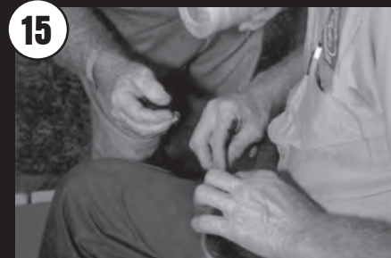
Insert strong cord into groove on the outside of vent rubber leaving long lengths at both ends for pulling.
